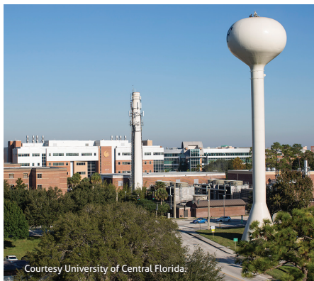
This 200,000-gal tower and an adjacent 100,000-gal storage tank regulate and store UCF's potable water supply.
