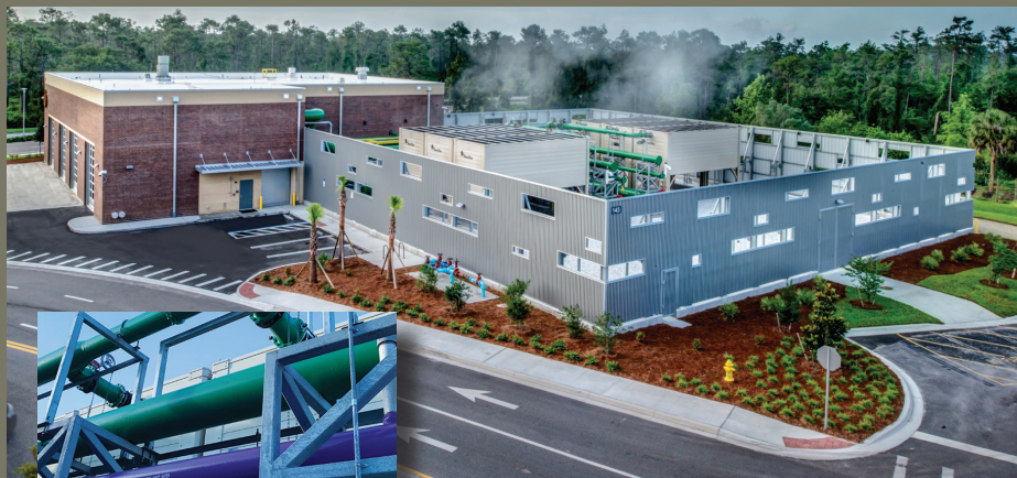
District Energy Plant IV.
